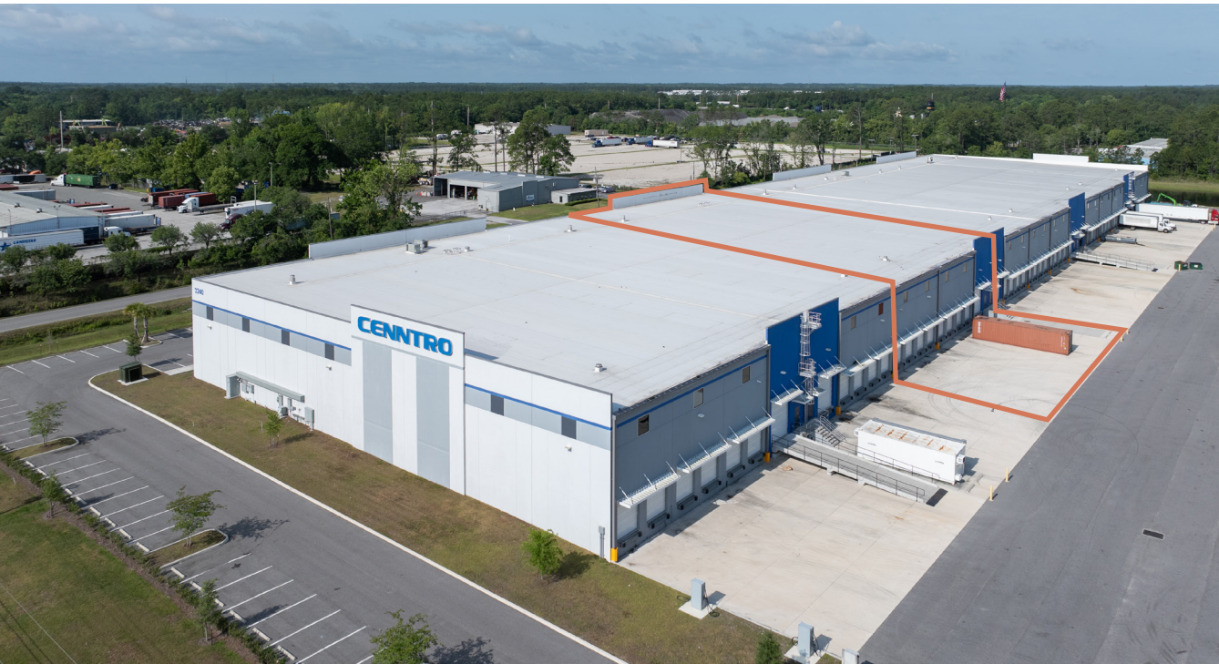
Photos | Suite 103: 50,000 SF (Demisable by 10,000 Bays)
