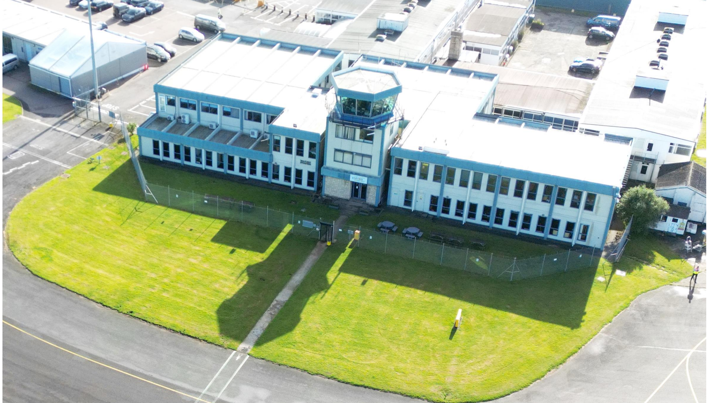
Main Yorkon Building (foreground) and Cherwell Blocks (to the rear)
