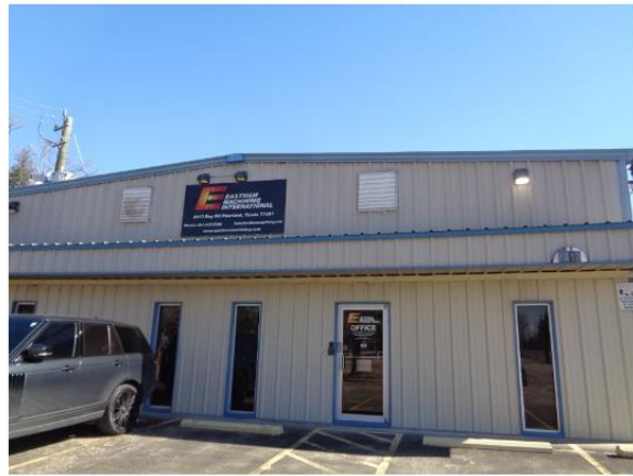
Exterior View of the Subject
