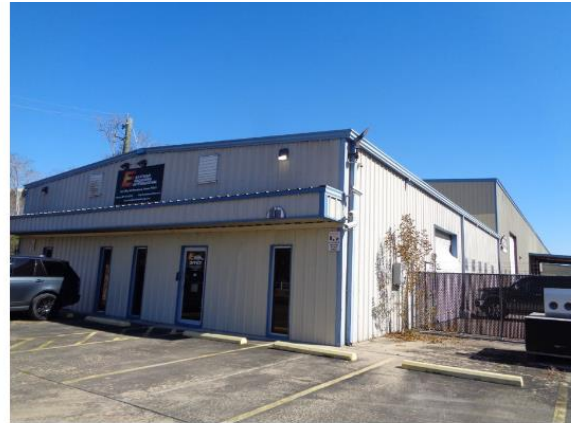
Exterior View of the Subject
