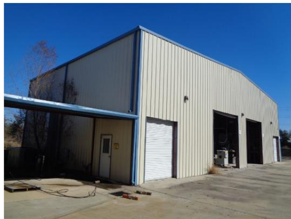
Exterior View of the Subject
