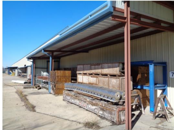
View of the Subject Canopy Area
