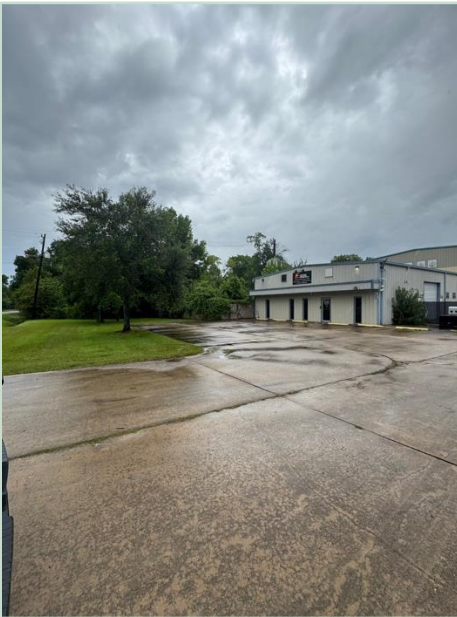
Office frontage & stabilized yard
