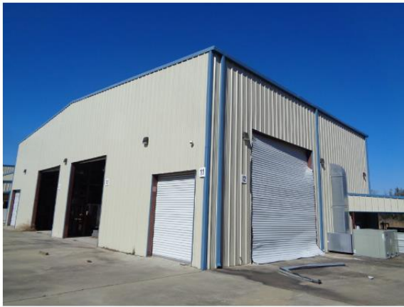
Exterior View of the Subject
