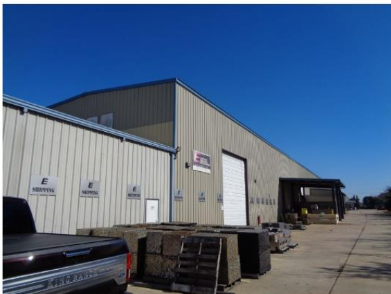
Exterior View of the Subject
