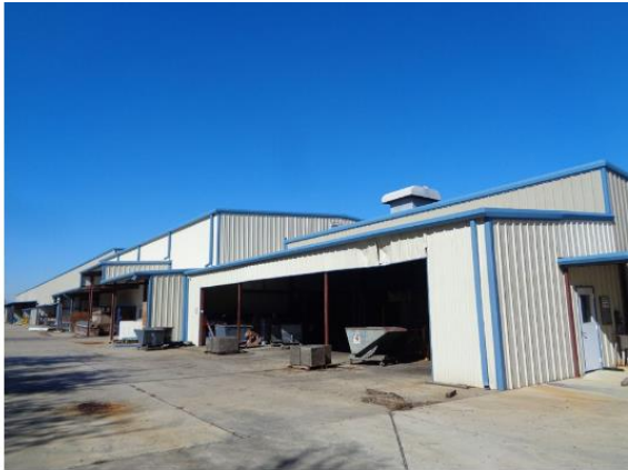
Exterior View of the Subject
