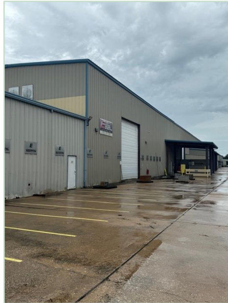
Shop elevation — loading & grade-level doors
