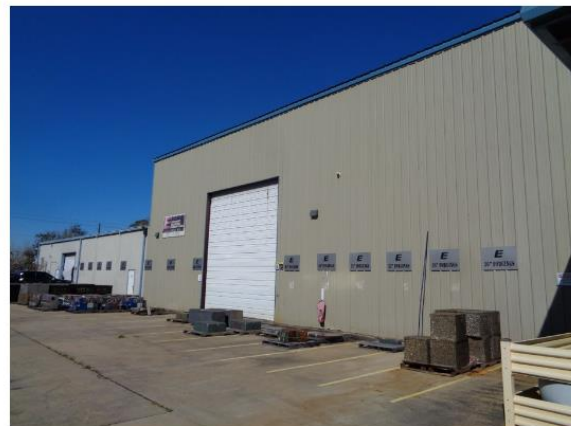
Exterior View of the Subject
