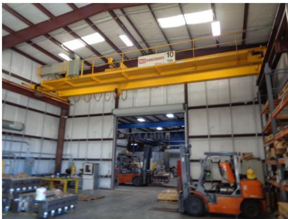
Interior View of the Subject
