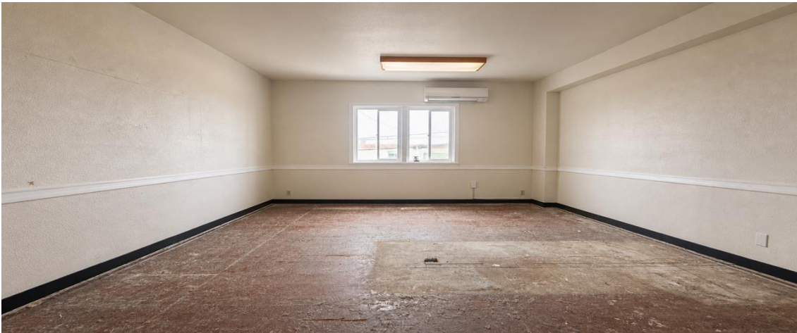
Private room / office with mini-split HVAC
