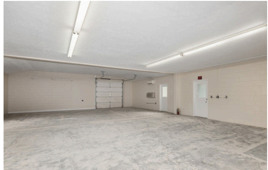
WAREHOUSE WITH ROLL UP DOOR
