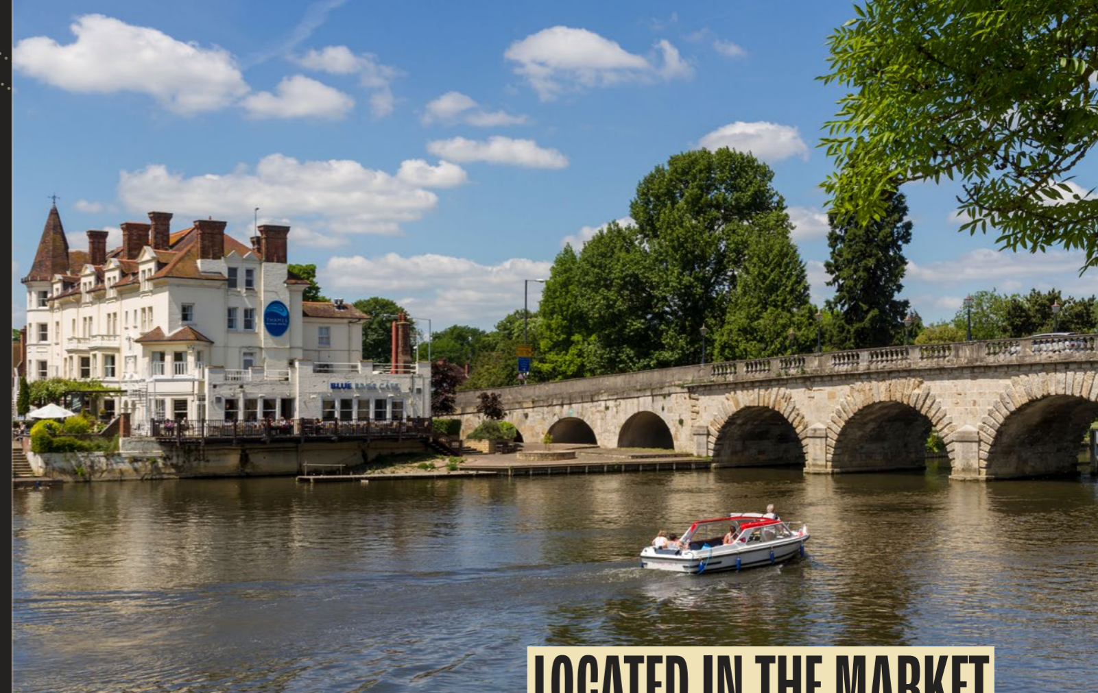
The Road Bridge over the river Thames
