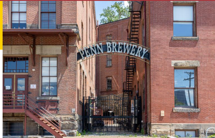
3 Story Office Building
