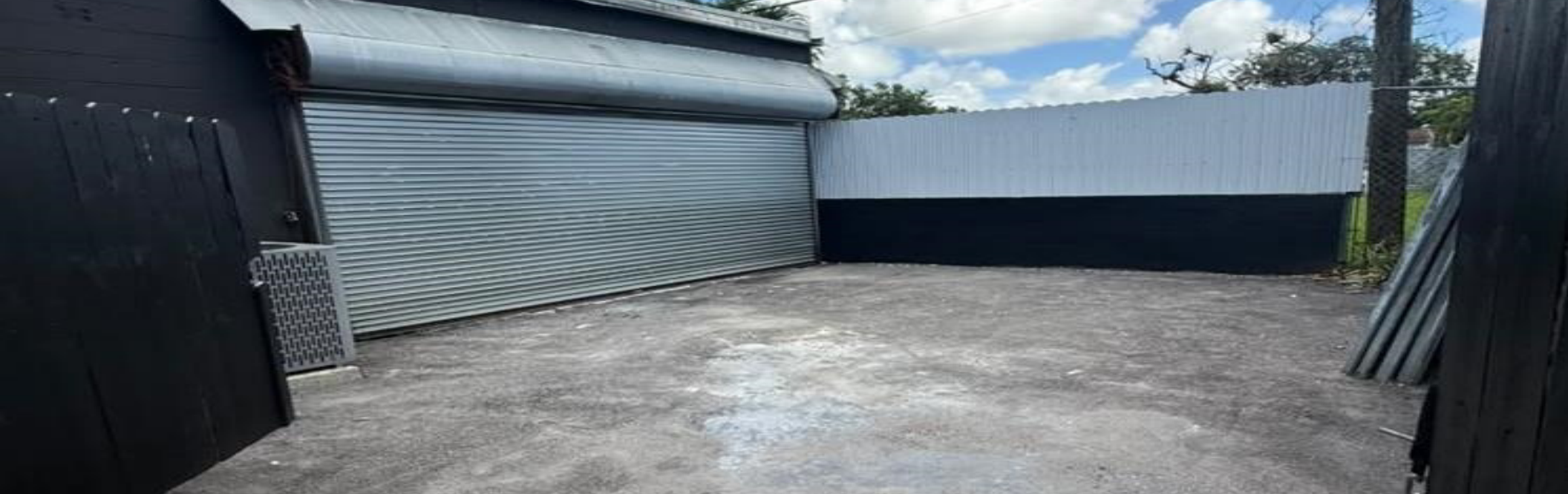
Rear Service Entrance
