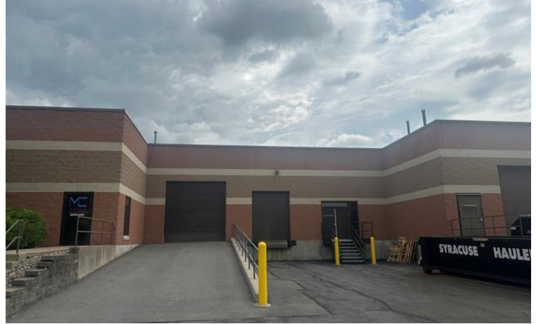
Loading Dock and Drive-in Door
