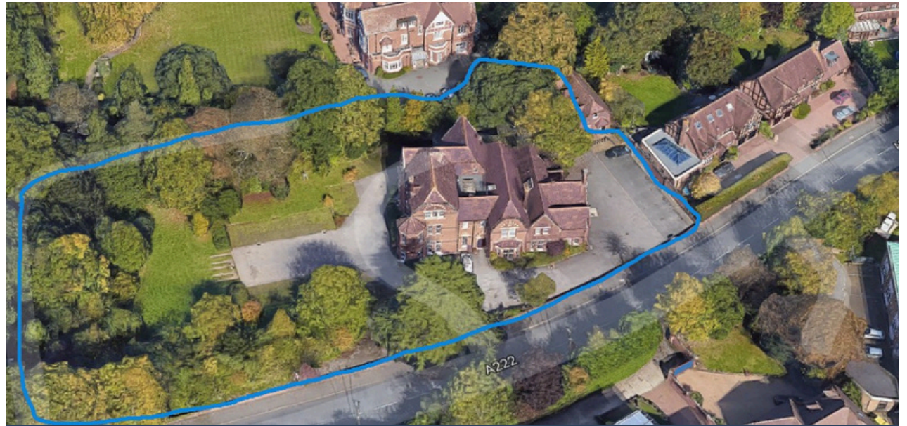
On Site Parking The building boasts a generous allocation of car park bays
