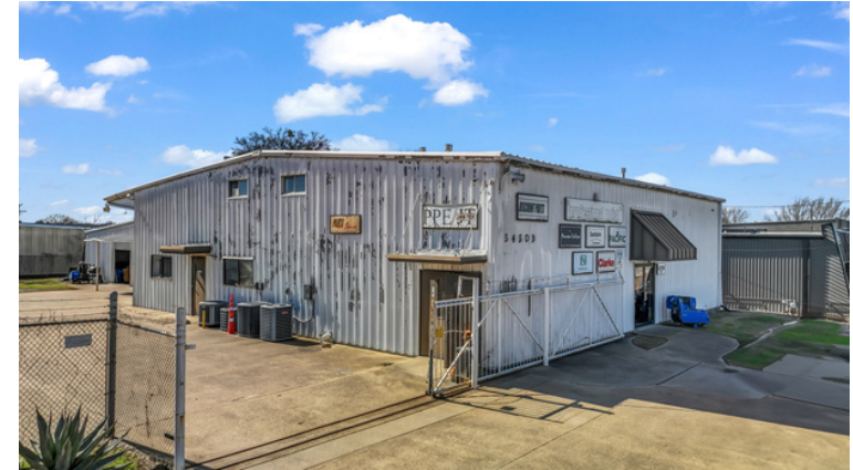
Functional light industrial building with flexible use potential.
