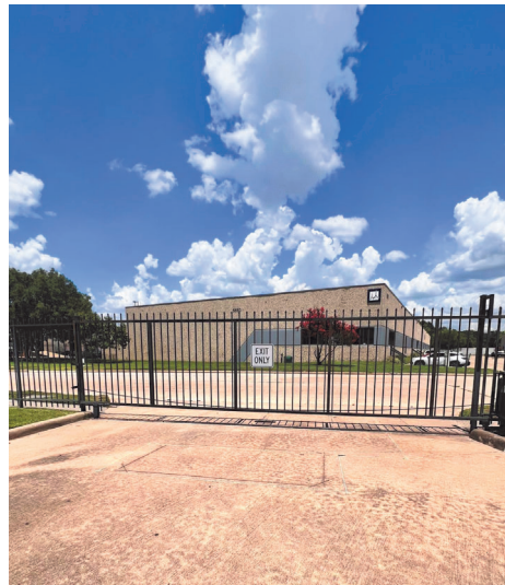
Private access control gate
