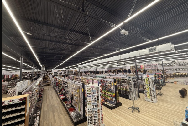
LED lighting throughout
