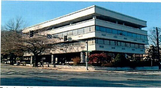
Exterior of Building
