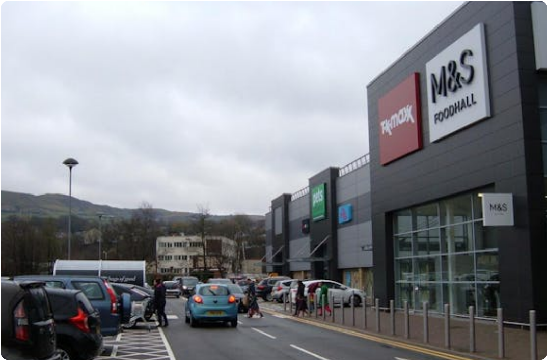
Building 5 New Hall Hey, New Hall Hey Road, Rossendale, BB4 6HL
