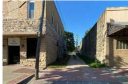
Center Street Alleyway Condition - Before
