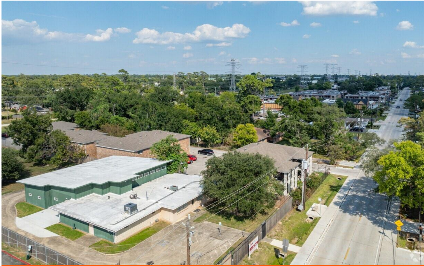
AERIAL — NORTHWEST CORRIDOR EXPOSURE
