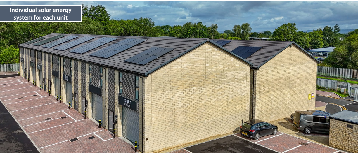
Plant room with 3-phase electric, DB board, water, solar control & BT fibre
