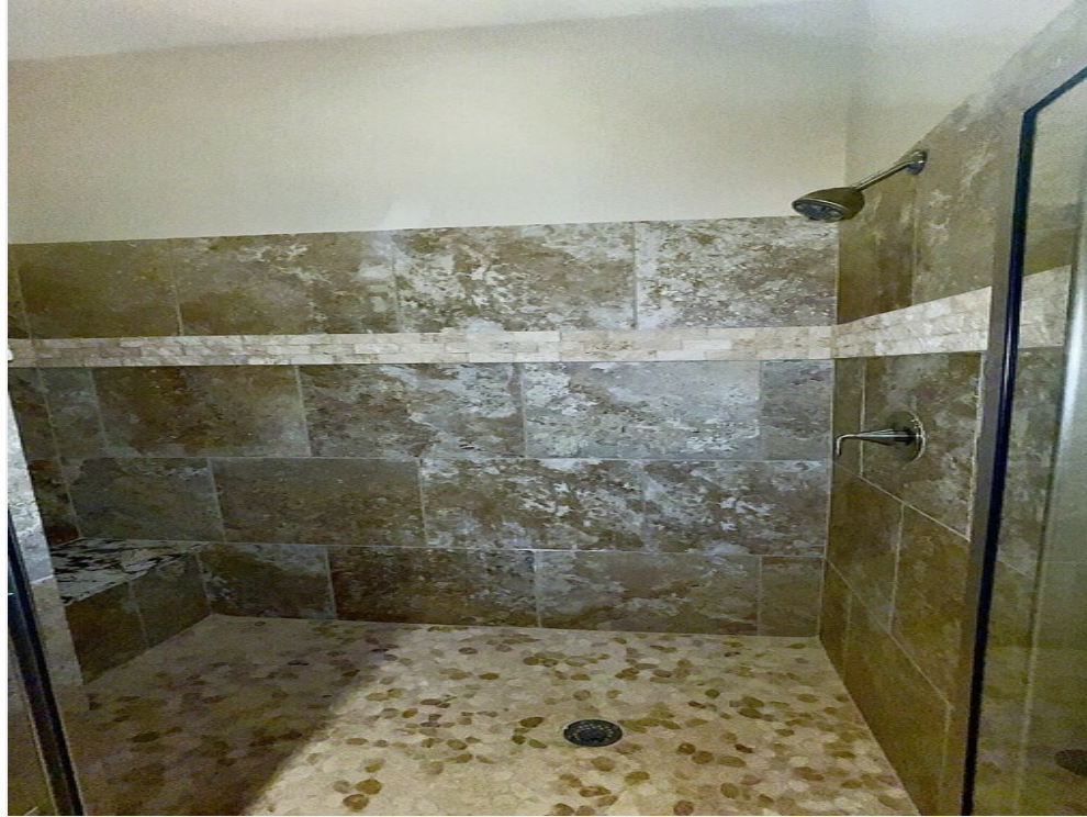
21555 Bathroom Between 2 Offices3
