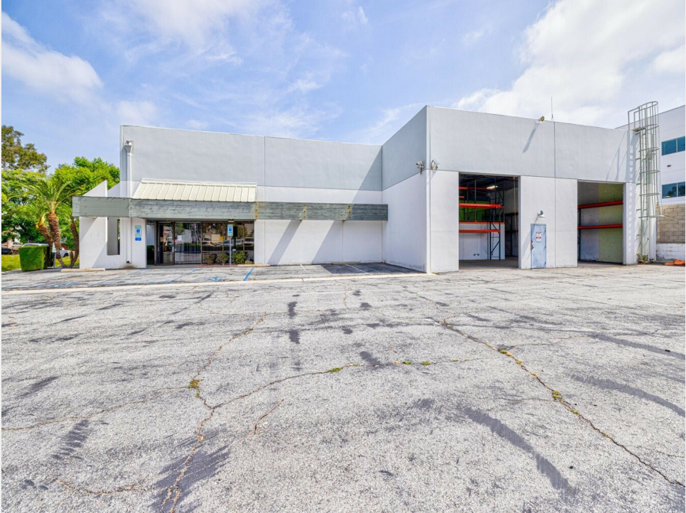
South Entry and Loading
