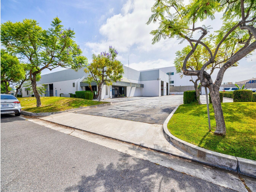
Front of Building
