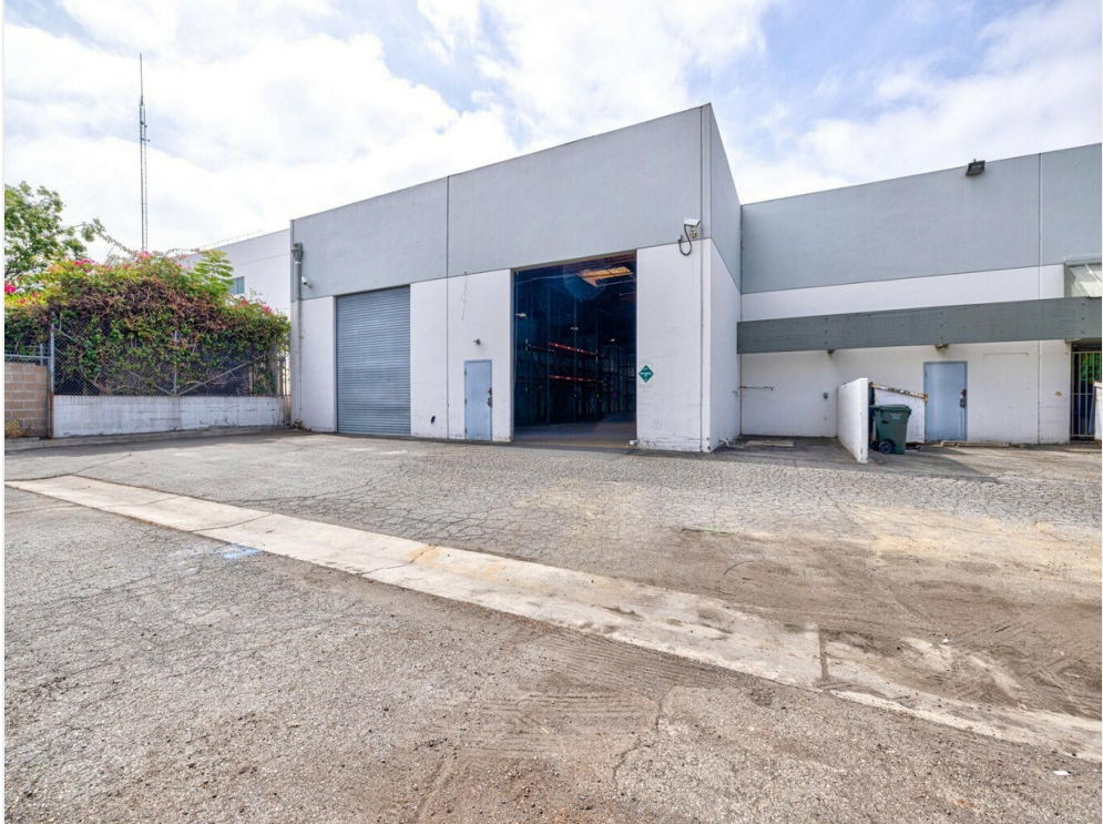
North Loading Doors
