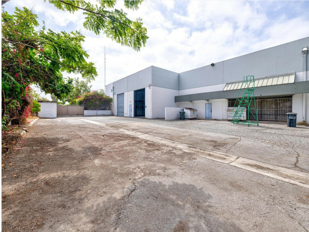
North Fenced Yard /Loading
