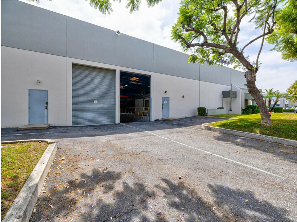
West Loading Dock Doors
