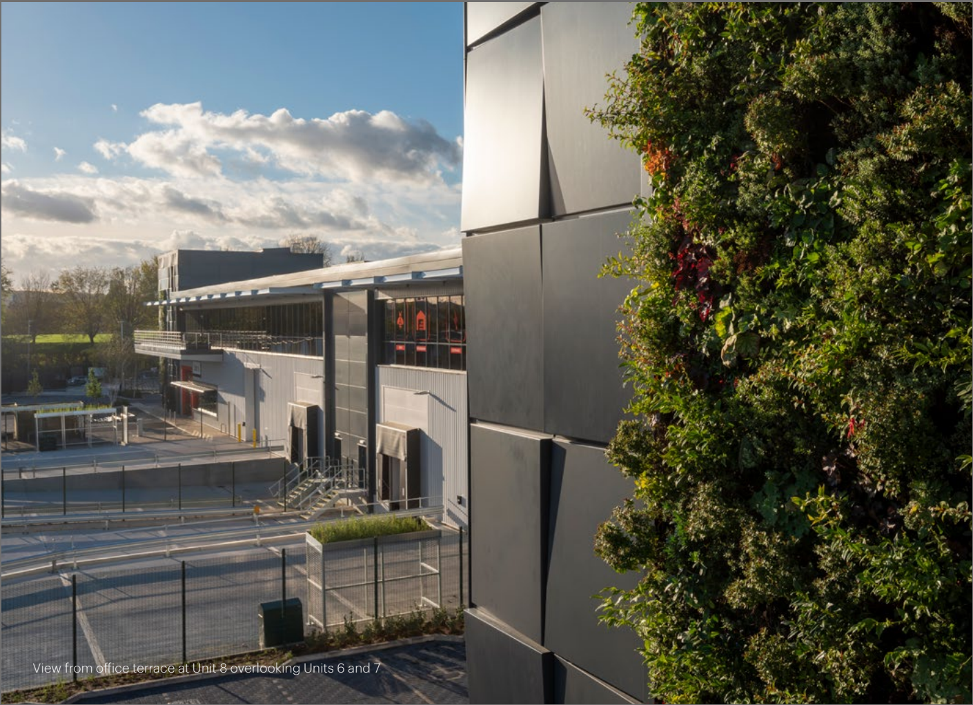
Image shows warehouse space at Unit 4
