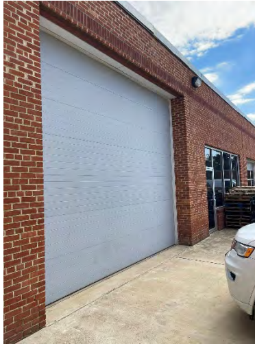
View of Drive-In Door
