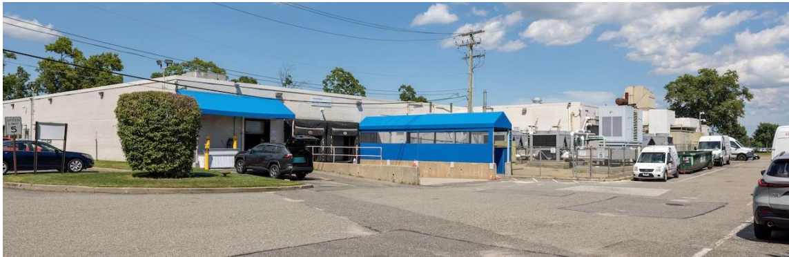
Covered service entry and mechanical yard.
