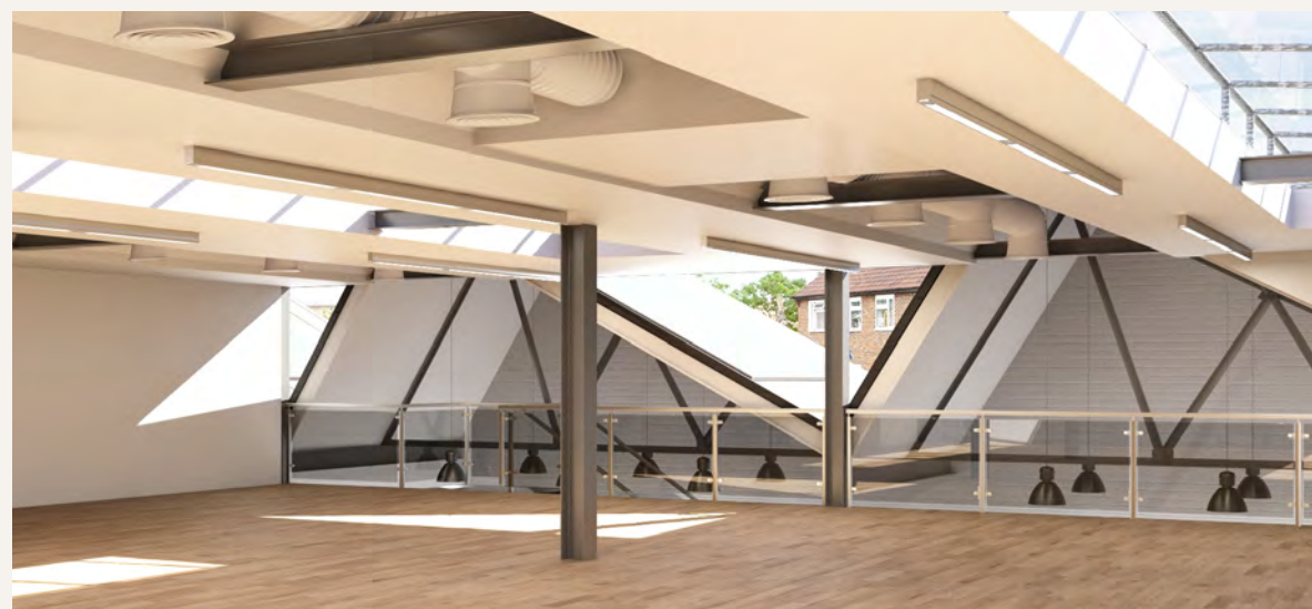
Kew Studios East - unit 1, mezzanine
