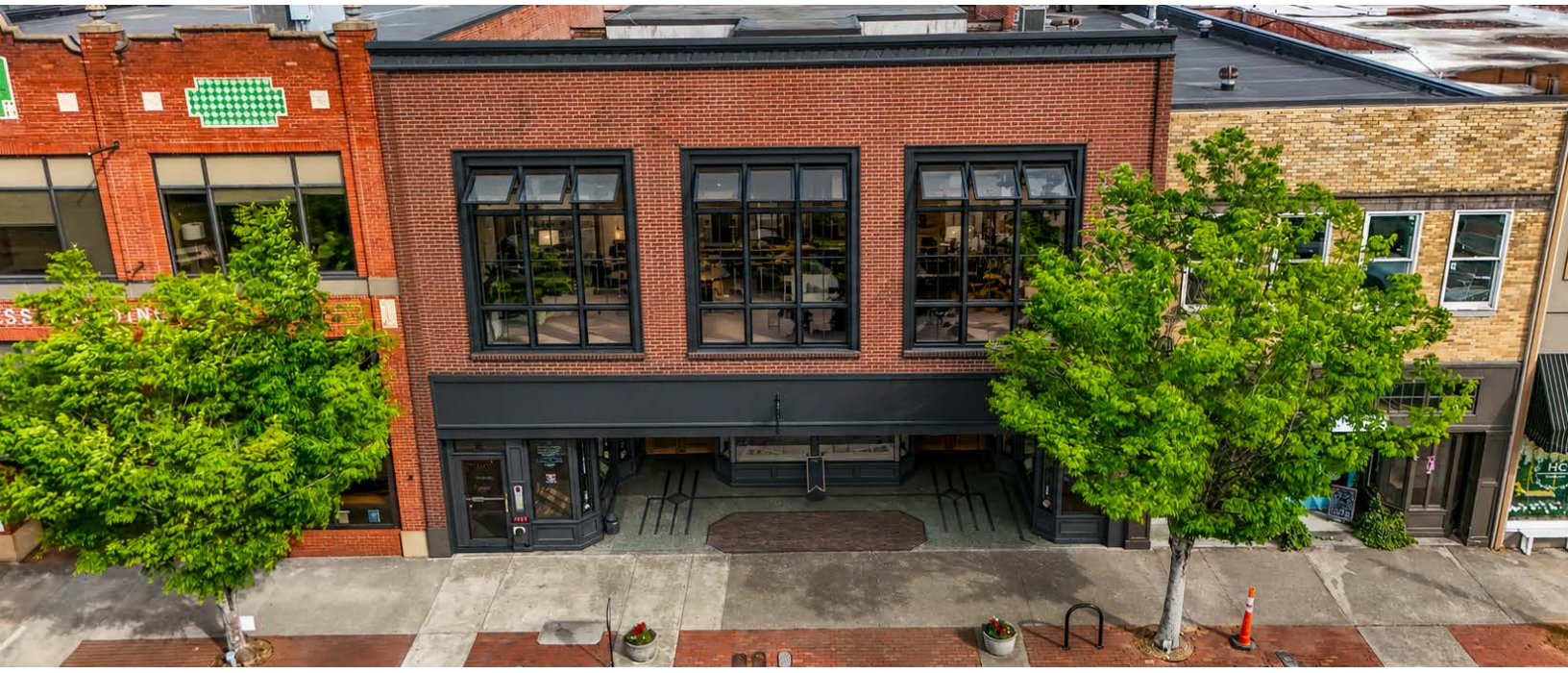
50% Facade Grant - Potential Renovation
