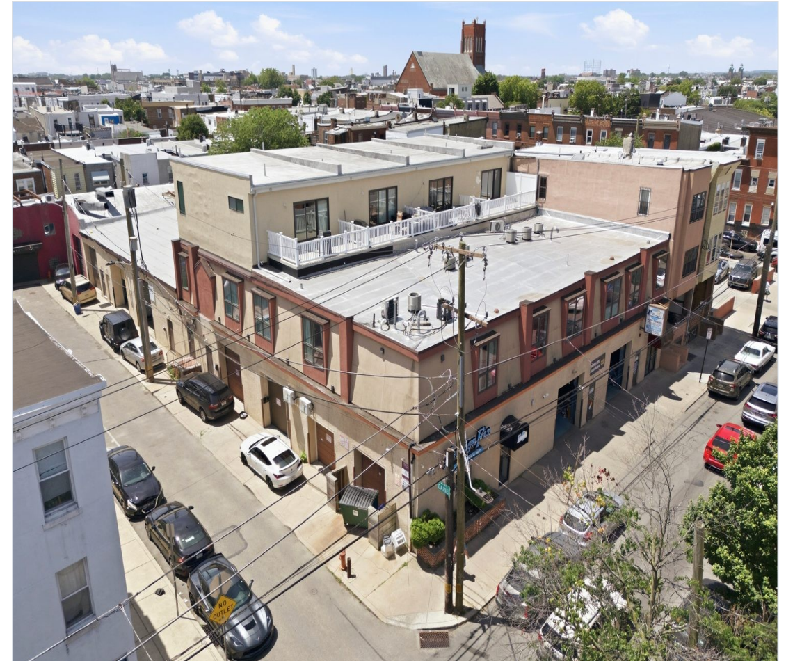
1400-1414 S Darien Street • East Passyunk Corridor
