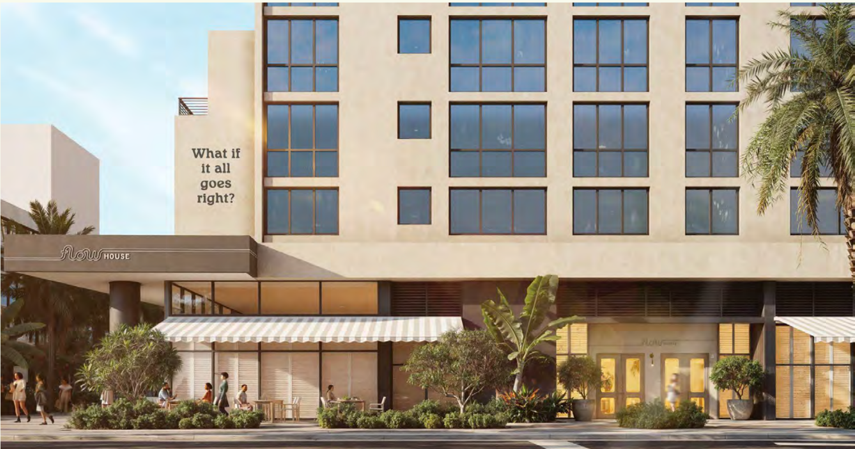
North Miami Avenue Facade
