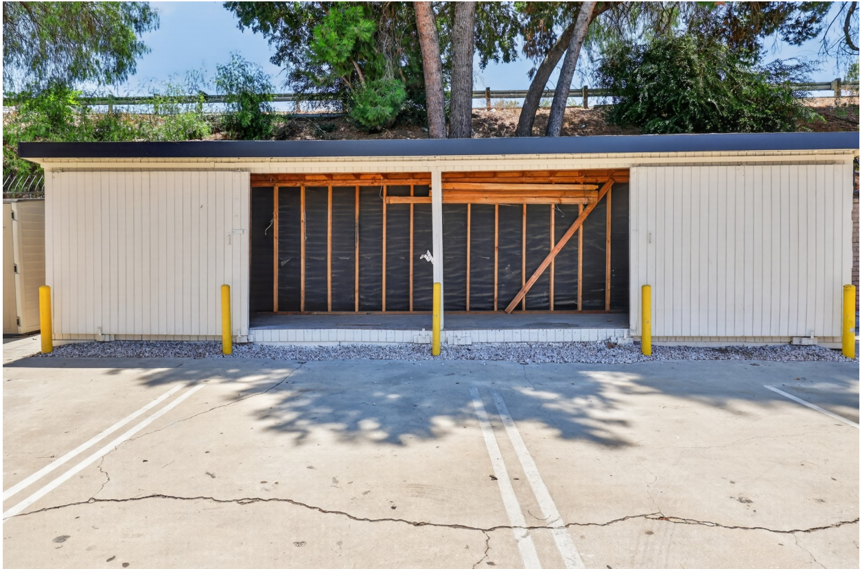
Additional storage area, framed and ready for build-out.
