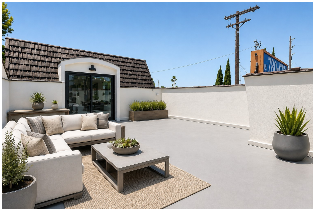
Second-floor usable deck, approximately 600 SF.
