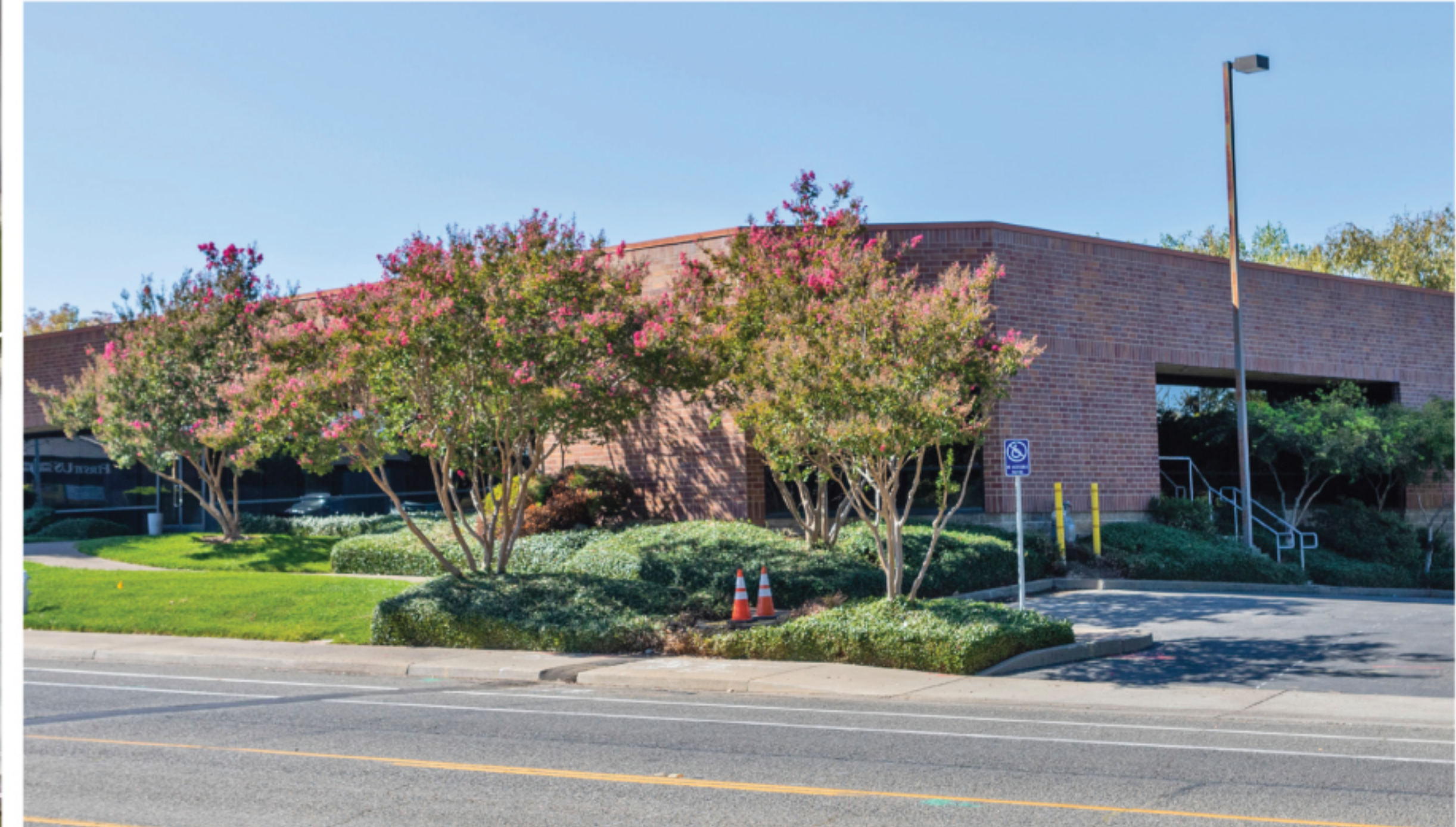
EAST SIDE OF THE PROPERTY
