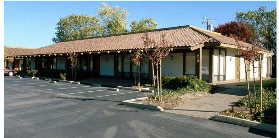
5 5723 Marconi Ave - Bldg 7 Carmichael, CA 95608
