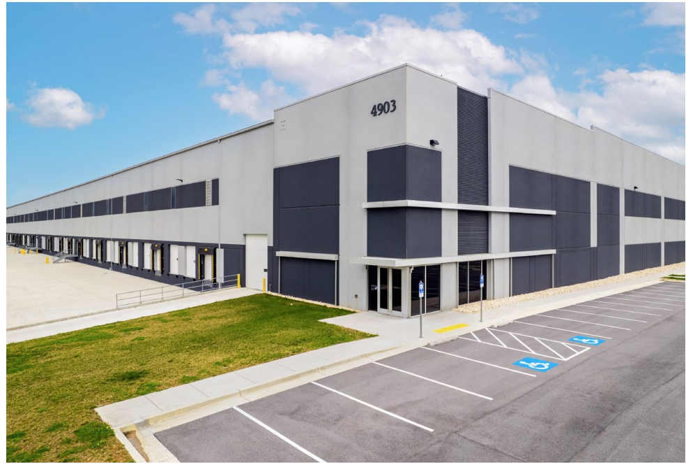
Building A | 365,400 sf | 4903 Winchester Avenue
