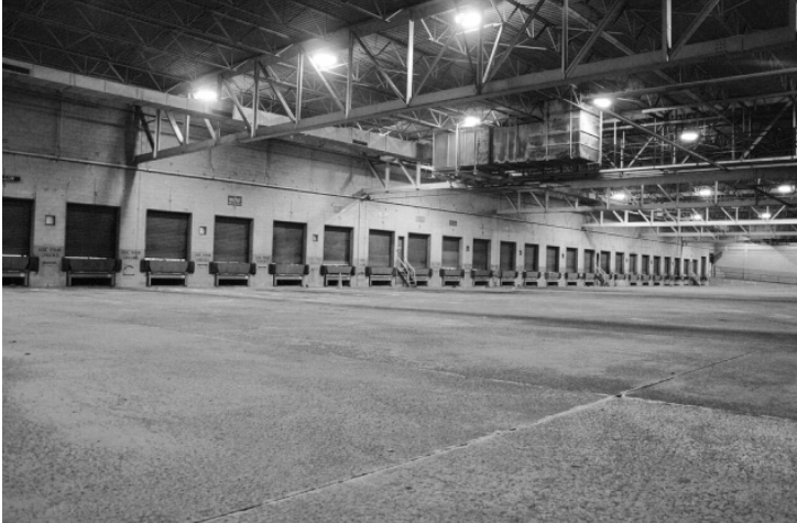
Interior Loading Docks
