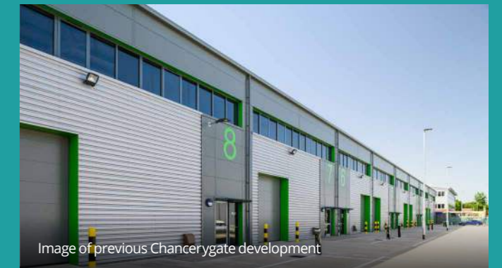
Image of previous Chancerygate development
