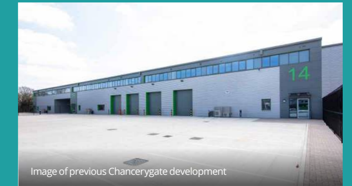
Image of previous Chancerygate development
