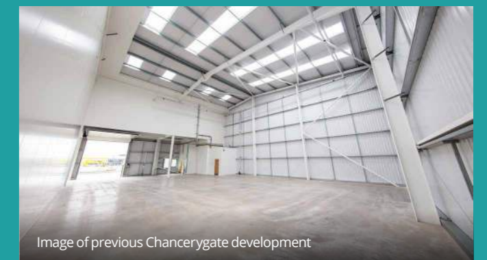
Image of previous Chancerygate development
