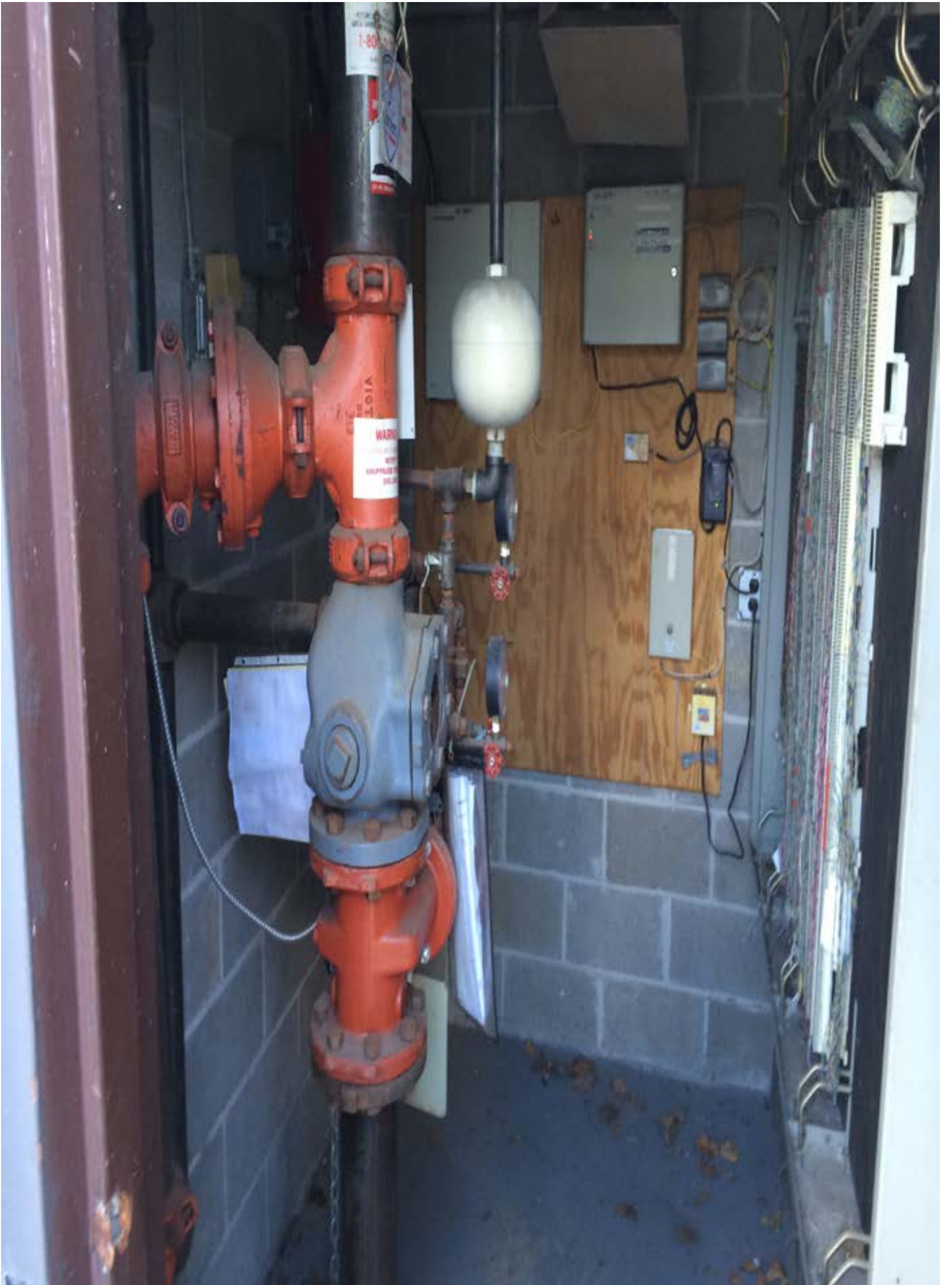
INSIDE SPRINKLER ROOM- INCLUDES ELECTRICAL PANEL
