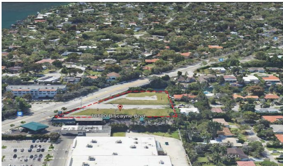
Looking south along Biscayne Blvd / canal
