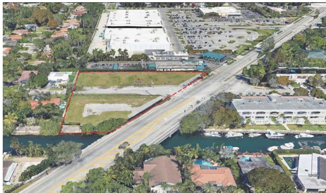
Looking north toward the site
