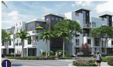
1 ATLANTIC CROSSING 777 East Atlantic Avenue
