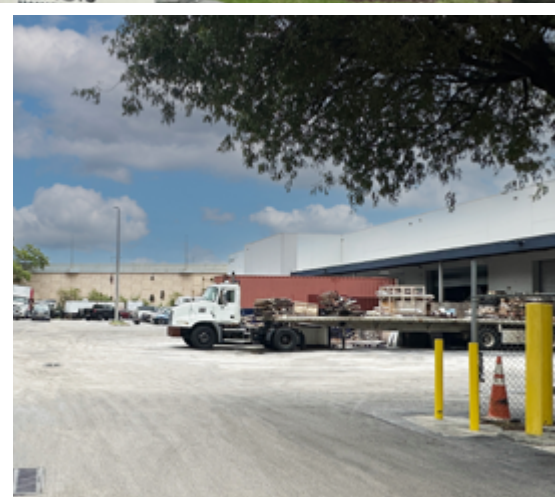
Secured truck court and parking
