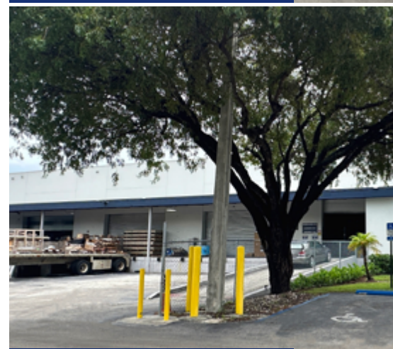
Oversized dock doors
