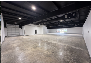
FINISHED WAREHOUSE BAY
