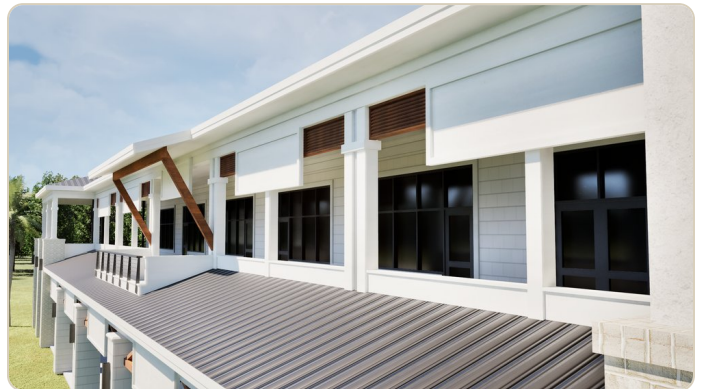
Second-floor covered walkway detail
