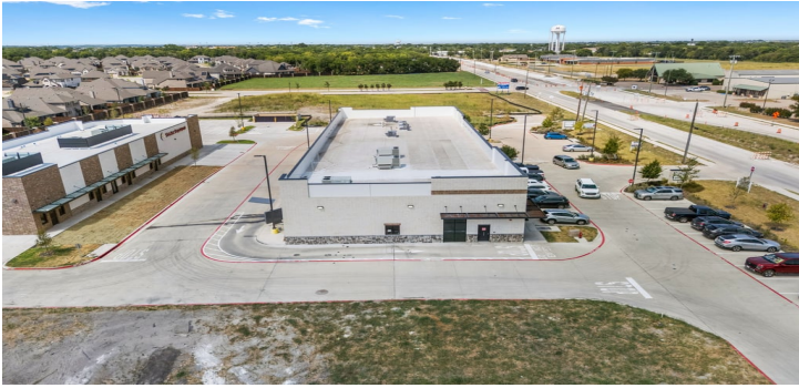
Monument Sign & Full Facade
