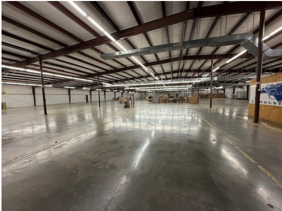
Conditioned Section — Polished Concrete, LED Lighting, 14'/17' Clear
