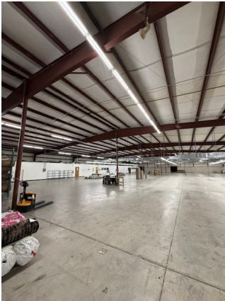
Conditioned Section — Steel Structure, Clean Walls, Dock Access
