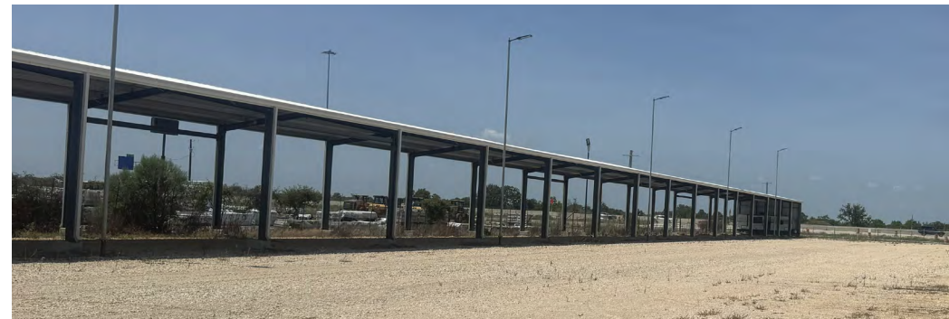
30' x 800' canopy structure
