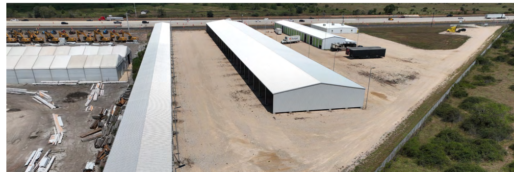
Large drive aisle
