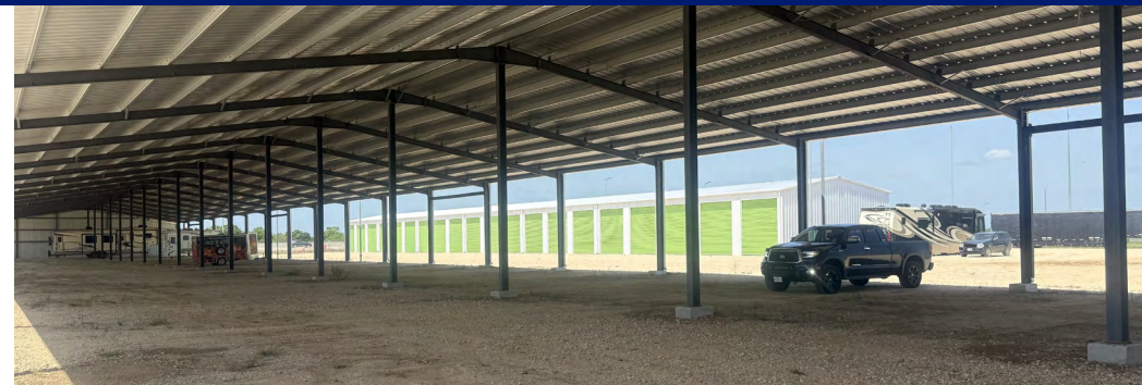
80' x 600' canopy structure
