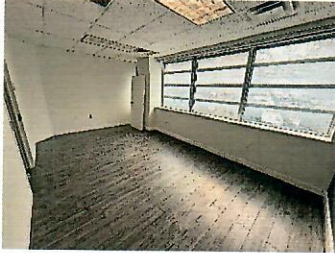
2 windowed offices facing Fenton St.
