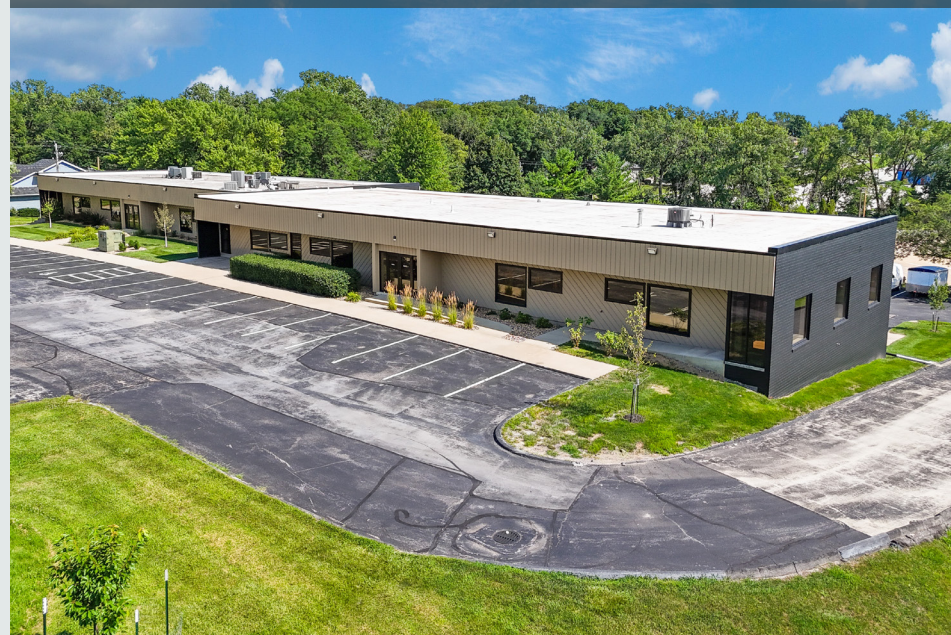
Upper Level - North Side
