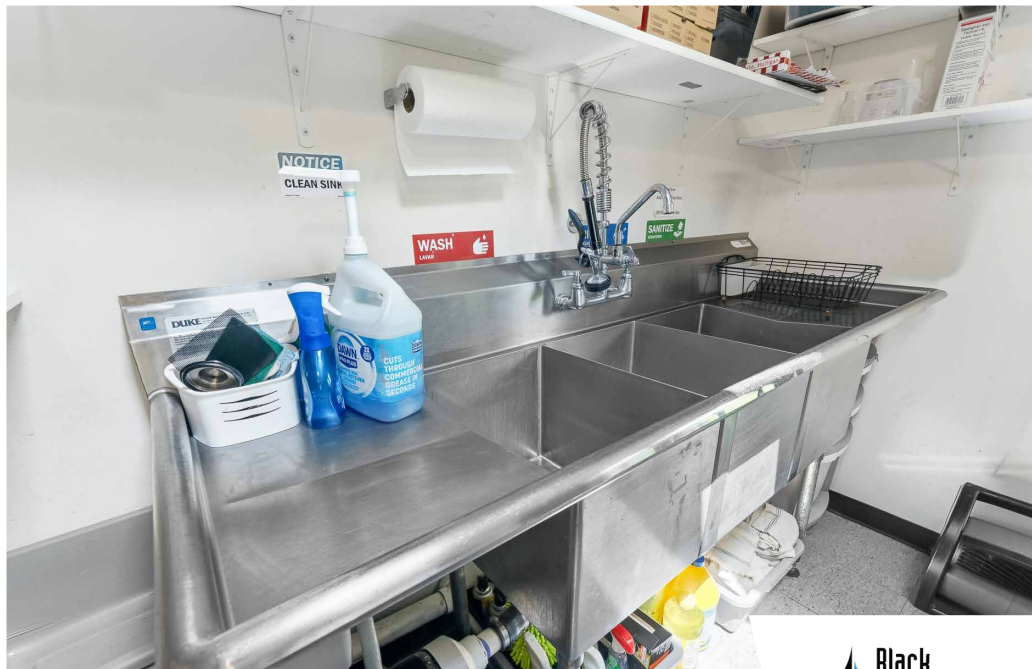
Restaurant Commercial Kitchen.
