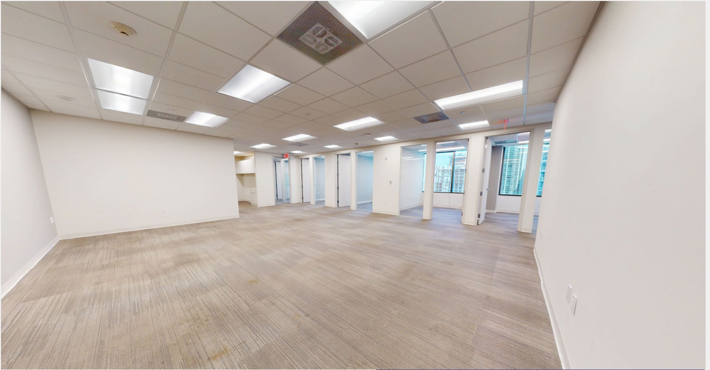
PERMITER OFFICES AND OPEN AREA
