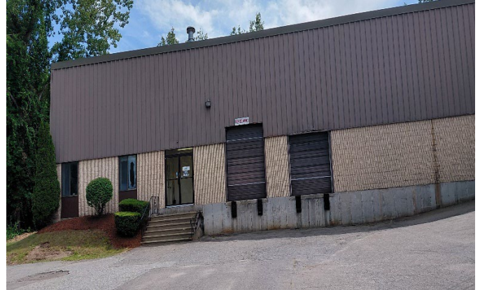
UNIT C LOADING
